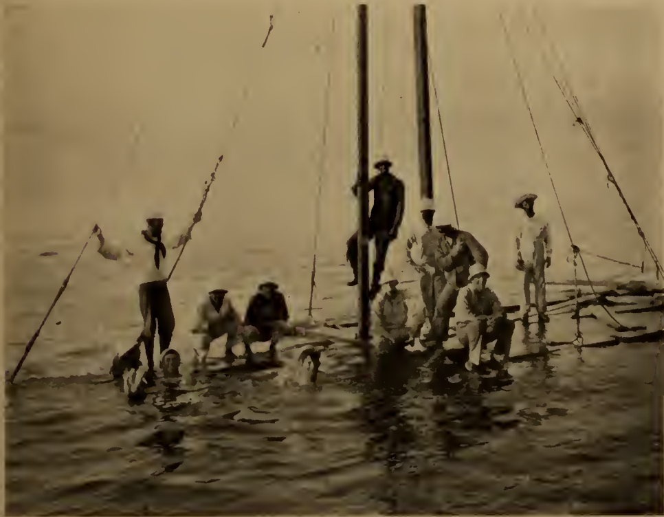
REPAIR CREW WAITING FOR A NEW TARGET.
